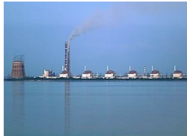
The six reactors from across the Kakhovka Reservoir, which supplies their cooling water
