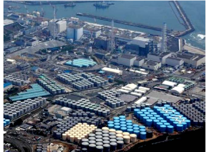
Some of 580 tanks being used to store the radioactive water.
