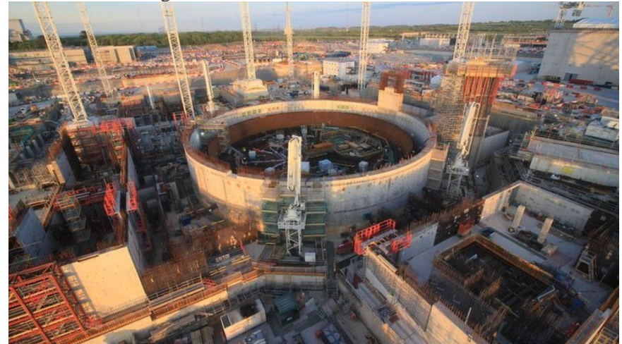
Recent photo of Hinkley Point C in construction
