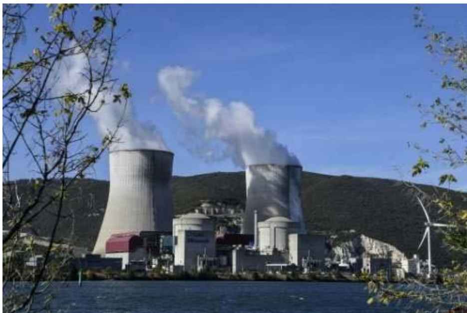
Cruas-Meyssas nuclear power plant
